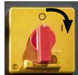
Switching on the main switch
